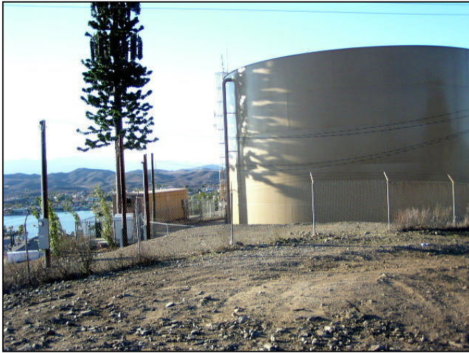
Photograph 5: View from Quail Valley candidate location, facing west.
