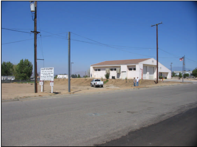
Photograph 1: View toward Menifee candidate location, facing northeast.
