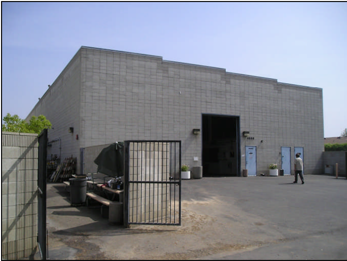
Photograph 3: View toward the Central Plant Building at 4090 County Circle Drive, facing north-northeast.
