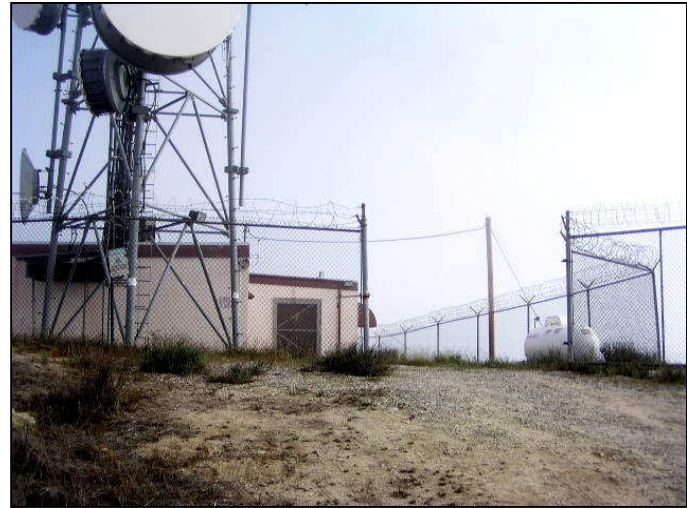
Photograph 4: View toward Box Springs candidate location, facing north.
