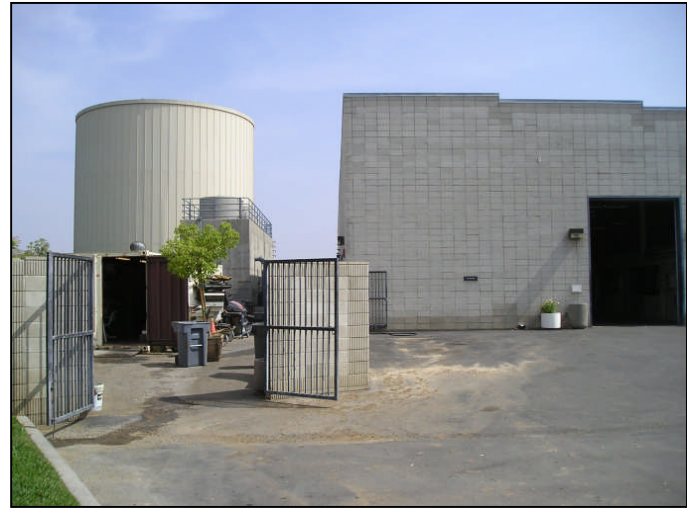
Photograph 4: View toward the Central Plant Building at 4090 County Circle Drive, facing north-northwest.
