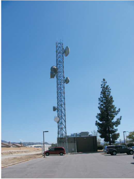
Typical communication tower in an urban setting (Existing county site in Hemet).
