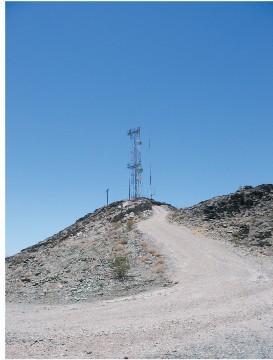
Typical communication tower in a rural setting (Existing county site west of Blythe).
